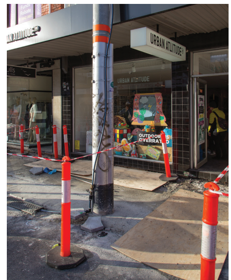
Temporary water supply secured to lamp post
